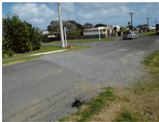
The area of recently tarsealed road which has since been dug up to put in a drainage pipe.
